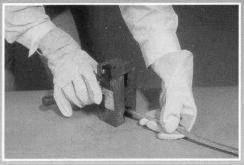
Clean the conductors and position them in the well dry mould.
